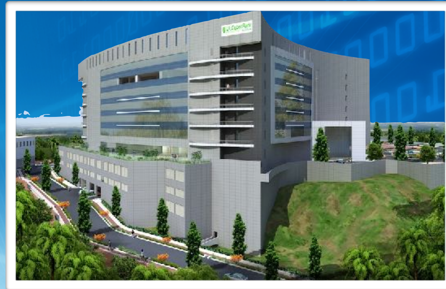
4.5 lakh sft structure completed
